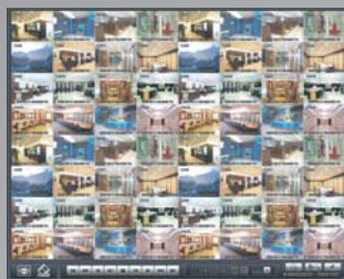
central monitoring system (CMS)
